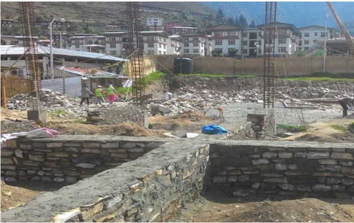
Changjiji community lhakhang construction
