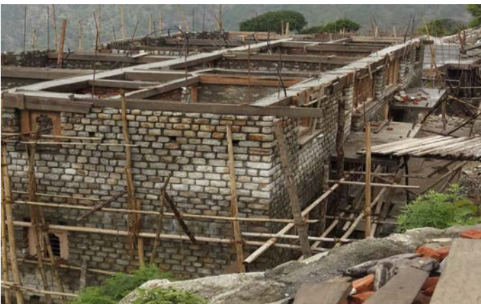
Lhuntse construction under progress
