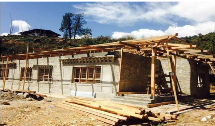
Gasa construction under progress
